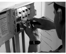
Installation is a snap with the roomy cabinet and horizontal terminal strips
